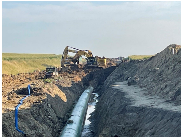
Facing north at MP 33.4, K&K backfilling trench north of County Road 8/154th Street
