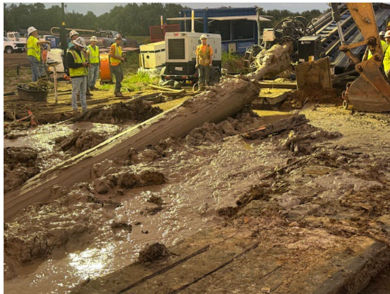
HDD P4-2 completed the pull
