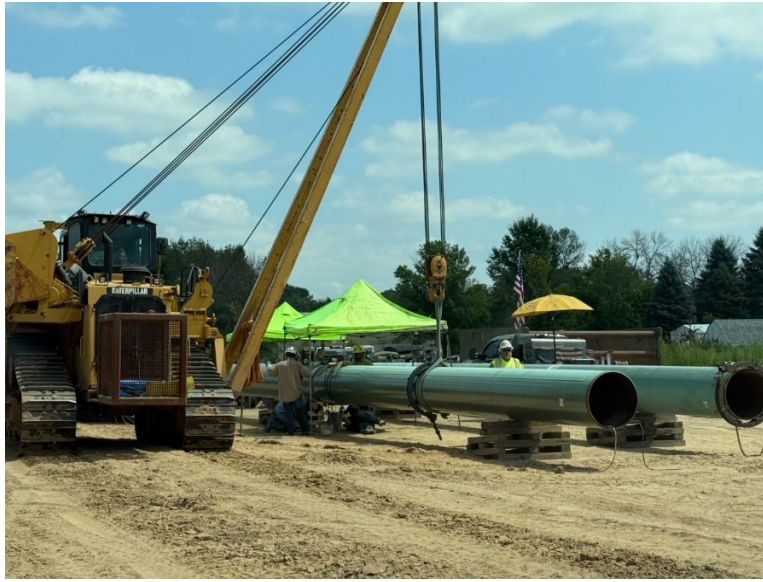
Facing west near MP 1.7, view of the contractor stringing and welding line pipe
