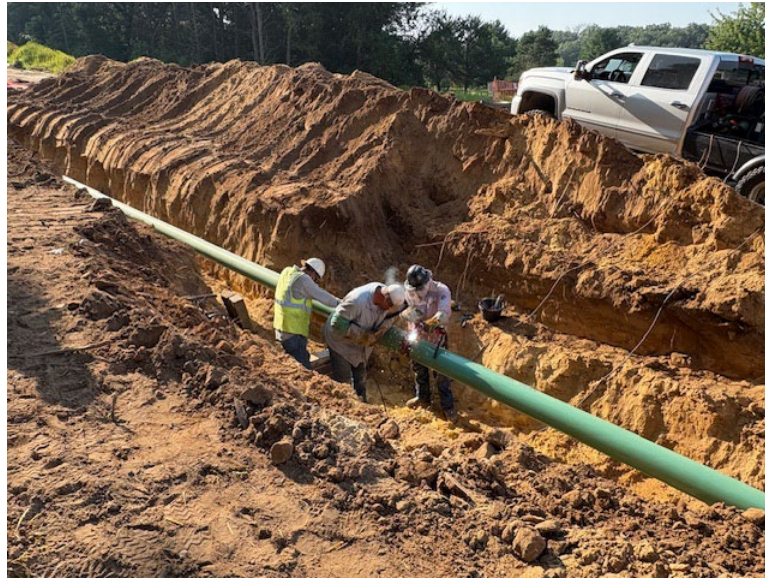
Facing south near MP 2.25, contractor performing tie-in
