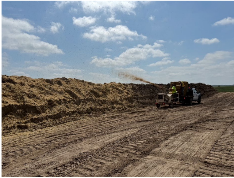
Facing south near MP 1.08, view of the contractor stabilizing the topsoil stockpiles
