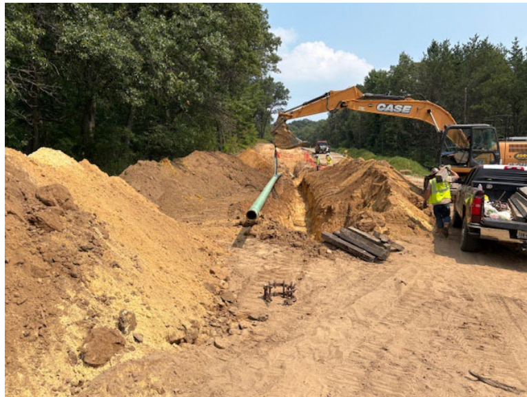
Facing east near MP 2.25, contractor lowering-in pipe
