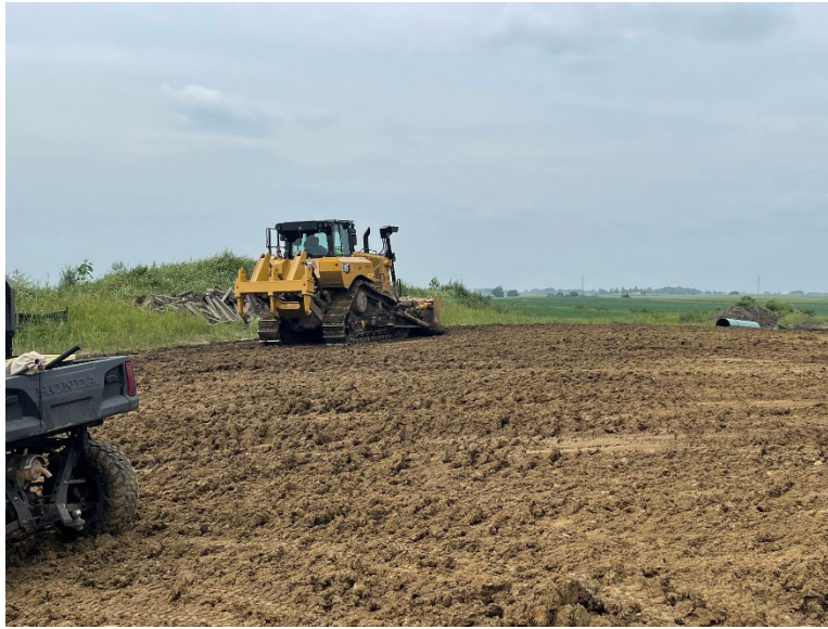
Facing south at MP 31.8, K&K restoring subsoil to grade south of 140th Street
