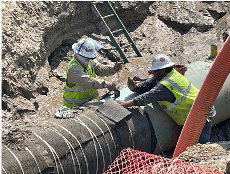
Facing southeast at MP 33.18, K&K installing test leads south of County Road 8/154th Street
