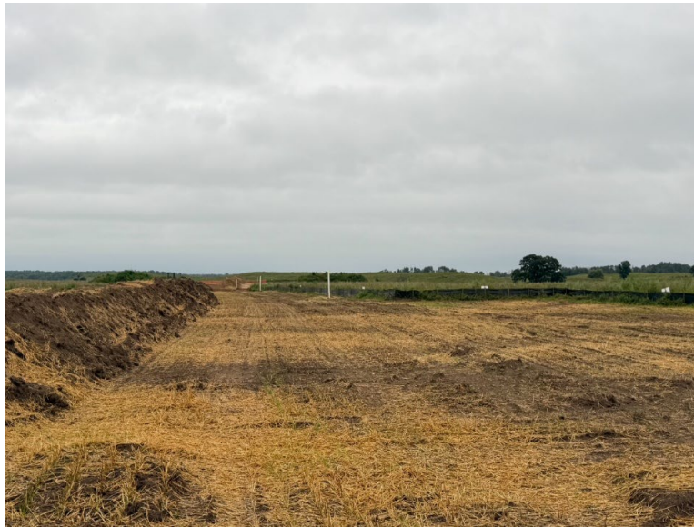
Facing south near MP 1.65, view of the ROW restored up to a travel lane, which is still required to allow access for final tie-in
