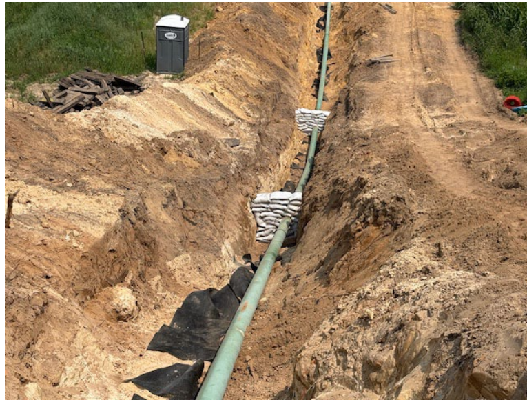
Facing east near MP 3.2, trench breaker installation
