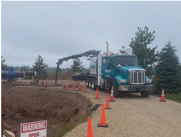
Facing south, Badger hydro vacuuming in the Hugo compressor station near MP 0.1
