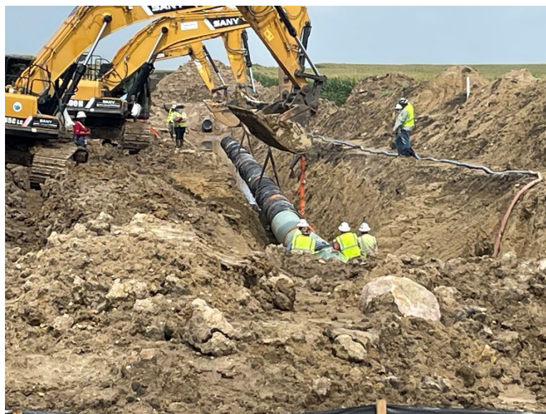
Facing north at MP 33.35, K&K lowering-in mainline pipe north of County Road 8/154th Street
