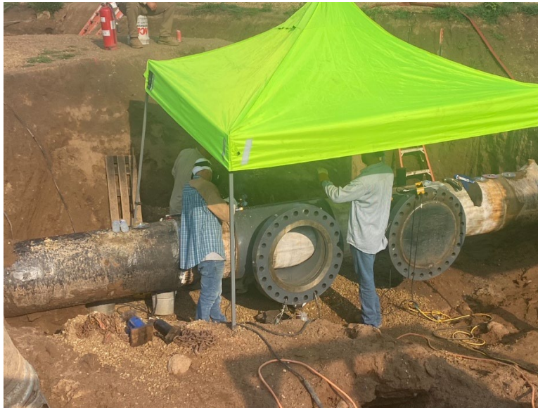
Facing south near MP 0.1, view of the contractor welding on the split tee in the Hugo compressor station
