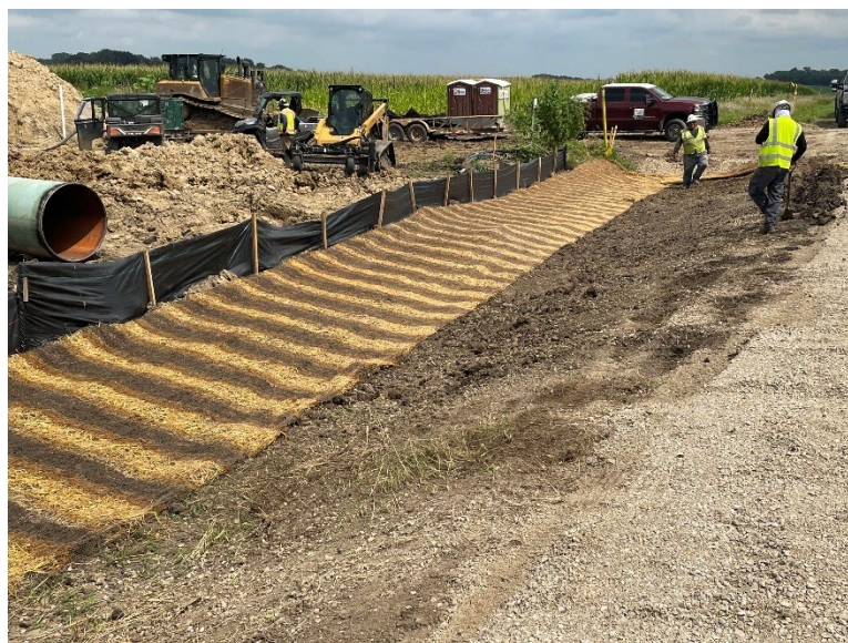
Facing east at MP 33.19, K&K installing erosion control blankets (ECBs) north of County Road 8/154th Street
