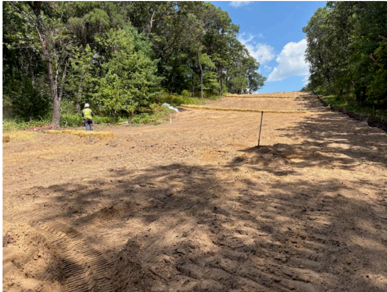
Facing east near MP 2.45, contractor installing slope breakers
