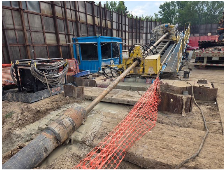
HDD P4-5 commenced the ream pass
